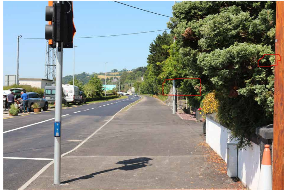
View 2 - from Johnstown Close looking westwards (1)
