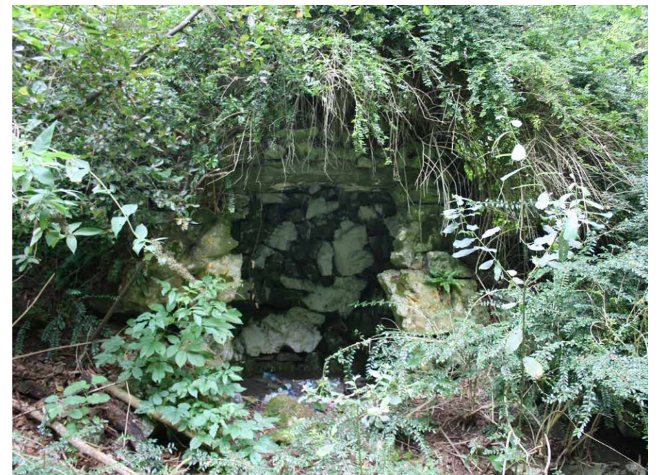
Existing Grotto - located within the lands south of 'The Terrace'
