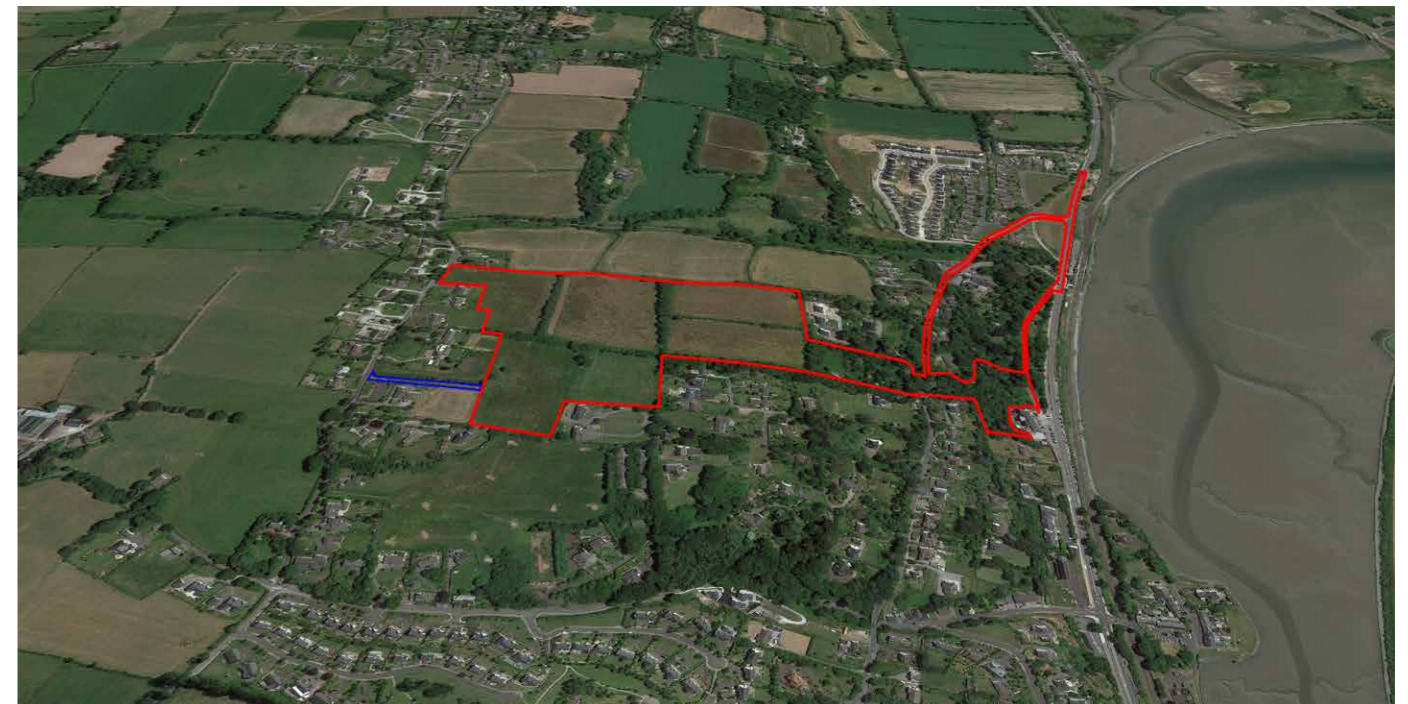
Aerial view from the west
