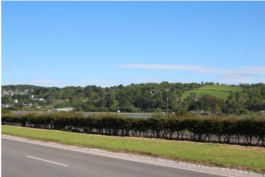
View 1 - from the N25 looking northwards at the subject site
